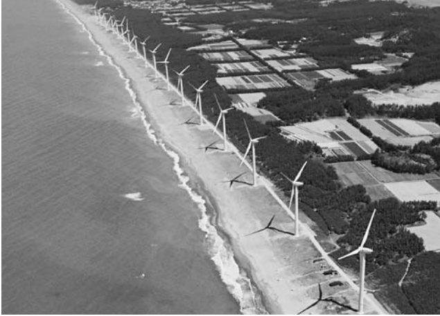
Fig. 6 Overall View of the Hachiryu Wind Farm At the Hachiryu Wind Farm, 17 units of 1.5MW wind turbine MD-77 are installed. MEICAPs have been tested in two wind turbines for demonstration test.
