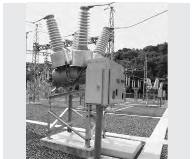
Fig. 9 72kV SF 6 Gasless VCB This figure shows an outside view of the VCB used on the Kyushu Shinkansen line. SF 6 gas-free design is used.
