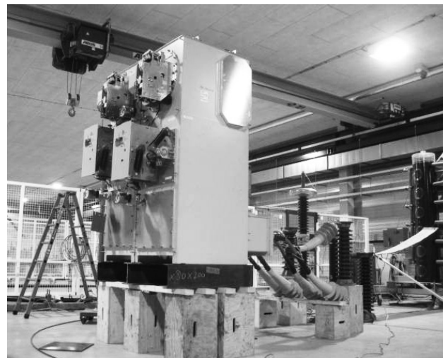
Fig. 5 A Testing Scene at the KEMA Testing Site (Withstanding Voltage Test)
