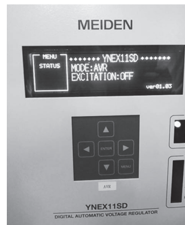
Fig. 1 Human Interface Part of Digital Type Static Excitation Control System
