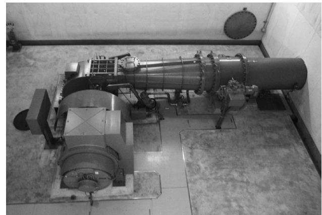
Fig. 3 Crossflow Water Turbine Generator
