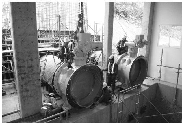
Fig. 5 Installation Work of the Inlet Valve
