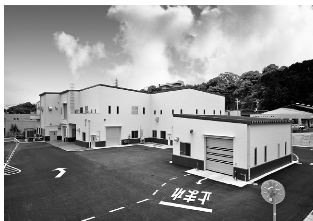
Fig. 6 Sludge Treatment Center
