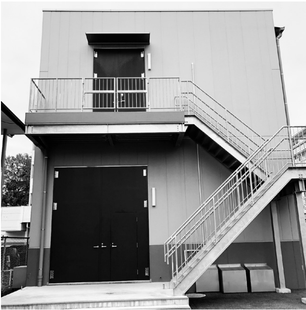
Fig. 2 Overall View of Traction Power Substation
